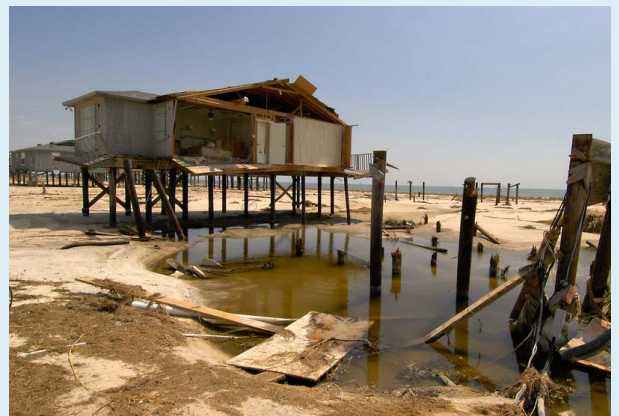
Hurricane Katrina's storm surge destroyed homes and roads on Dauphin Island in 2005. Credit: FEMA.
