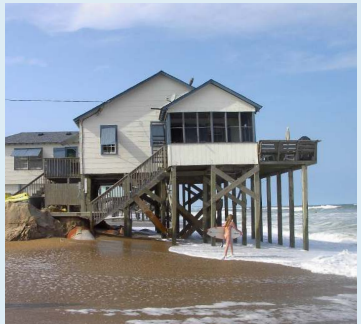
Beach houses in Nags Head are vulnerable to severe storms, flooding, and coastal erosion. © James G Titus; used by permission.
