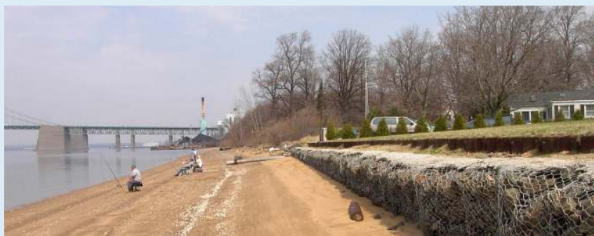
This beach in Pennsville along the Delaware River could be lost as sea level rises, if the shore erodes up to the shore protection wall to the right. © James G. Titus; used by permission.
