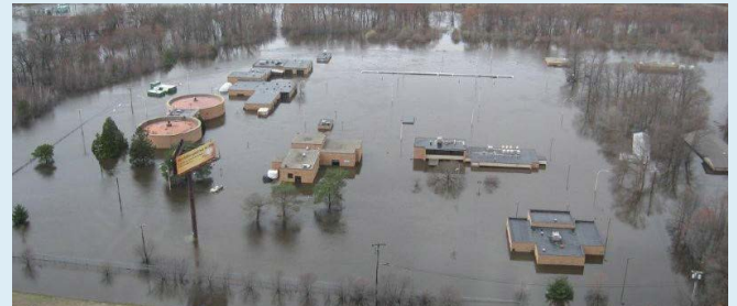
Historically heavy rains in spring 2010 caused the Pawtuxet River to flood the Warwick wastewater treatment plant (shown here) and many homes and businesses. Credit: Warwick Sewer Authority.
